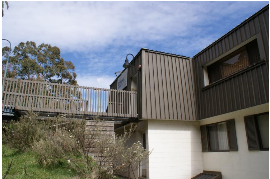
Figure 10: Photo of the Southern side of the building and elevated walkway
