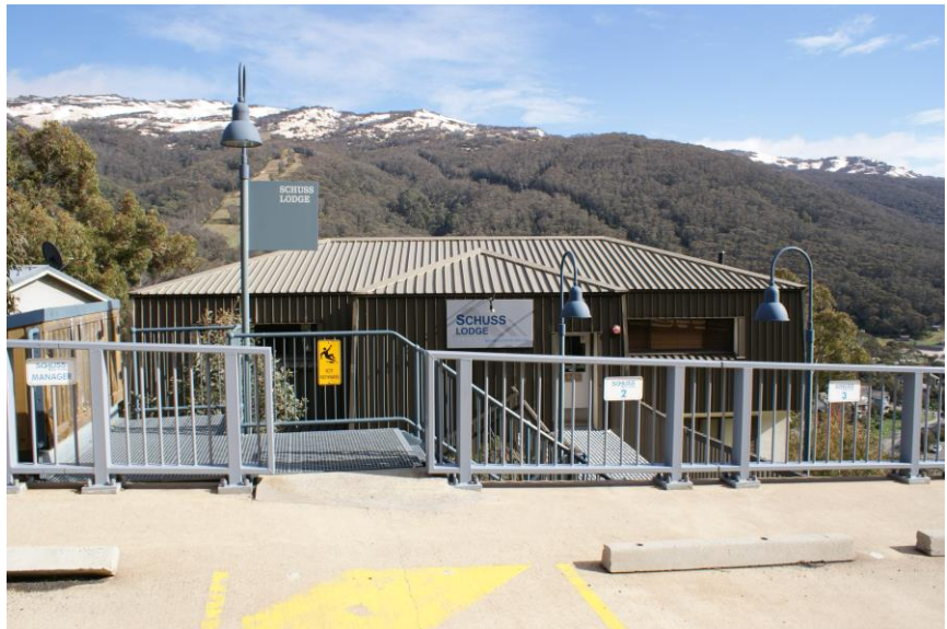
Figure 5: Photo of the southern elevation of the building from the car park on the edge of the Alpine Way
