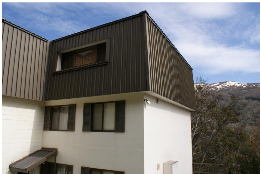
Figure 9: Photo of the proposed southern cantilevered additions on Level 4 (top floor)
